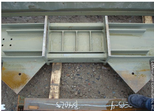
▲ A sample shear link at Dudley Square.
