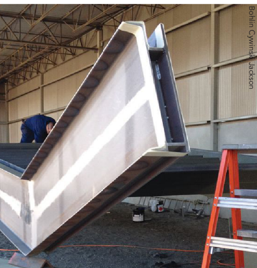
▲▼ The 10-ft, 6-in.-wide feature stair rises 29 ft between levels 1 and 3 and runs 93 ft continuously along the atrium.
