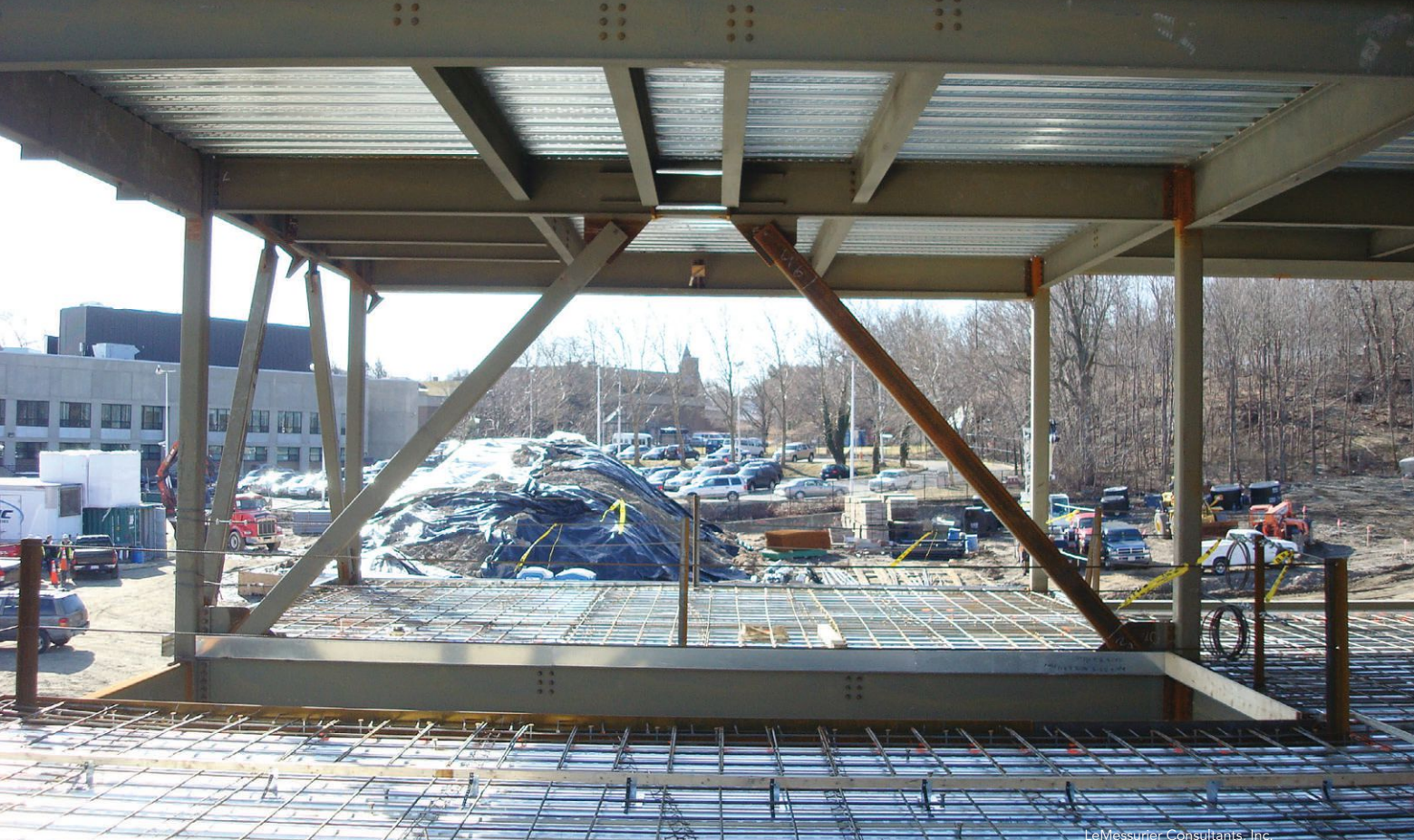
▲ Throughout Dudley Square Police Station, uniformly sized HSS column sections were designed to be exposed to view.
