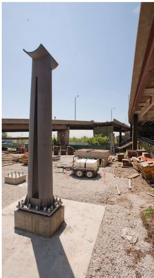
▲ ▼ The flyover spine is supported by steel columns created from 1¼-in. steel plate bent into a 30-in. by 22-in. elliptical shape along the main alignment and by cantilevered concrete abutments at its ends. At three locations, the path is supported directly from the existing bents of Lake Shore Drive.
