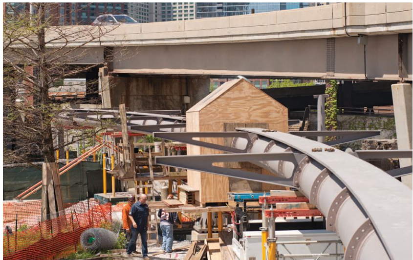
◀ ▶ ▼ The 1,750-ft-long, $60 million “Navy Pier Flyover,” now under construction as part of Mayor Rahm Emanuel’s “Building a New Chicago” program, will eventually relieve congestion along the most heavily used section of the 18.5-mile Lakefront Trail.
