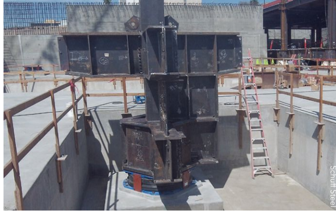
▲ A steel assembly atop one of the seismic isolation devices.
