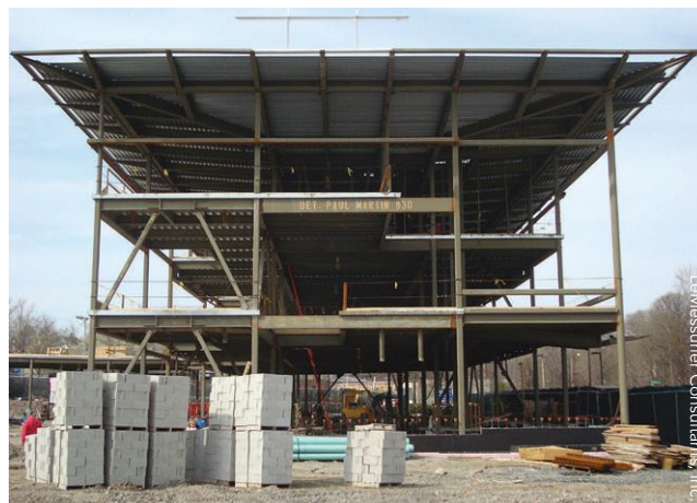
▲ The 8-in.-square HSS columns provided adequate capacity in most cases under load combinations.
